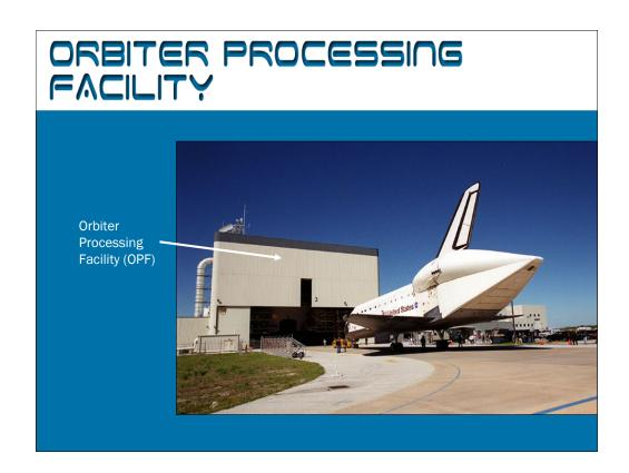
The orbiter is processed at one of three Orbiter Processing Facilities at KSC after landing and before rolling to the VAB for stacking. At the OPF, the orbiter is prepared for it's next flight. The Payload may be installed horizontally at the OPF or vertically at the launch pad.
